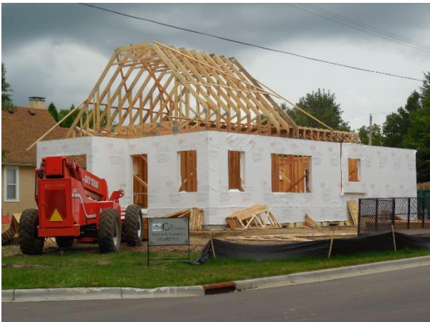
Under Construction Single-Family
