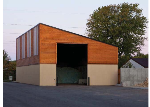
Public Works Salt Storage Facility
