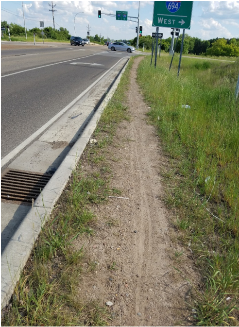
The desire path present along State Highway 120 (Century Avenue), just north of I-694, is a strong indicator for the need to improve bike and pedestrian facilities. This frequently used path is a critical connection between White Bear Lake and communities south of the freeway.
