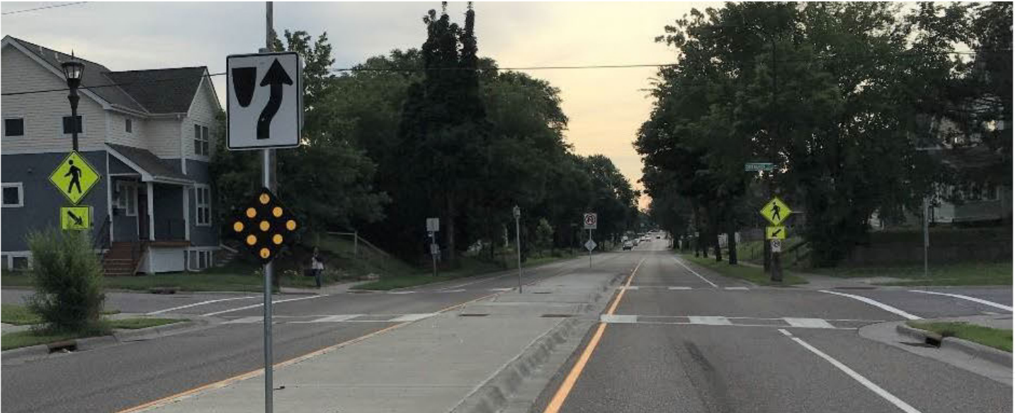
Median treatment to facilitate two-stage crossing and provide pedestrian refuge on a four-to-three lane conversion of Maryland Avenue at Greenbriar Street in Saint Paul, MN.
