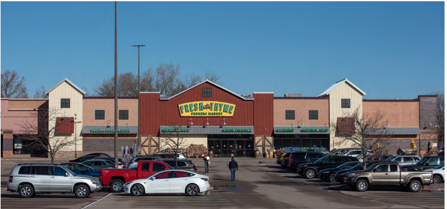
Shopping center at County Rd E and I-35E
