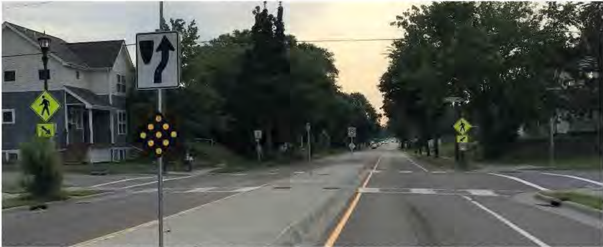
Median treatment to facilitate two-stage crossing and provide pedestrian refuge on a four-to-three lane conversion of Maryland Avenue at Greenbriar Street in Saint Paul, MN.
