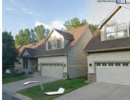
Townhouses at Hidden Lake Point, at 694 and Century Ave
