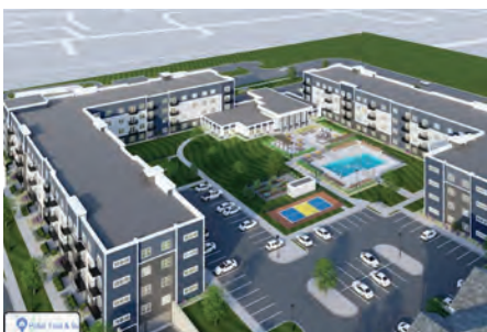
The Lochner, currently under construction.
