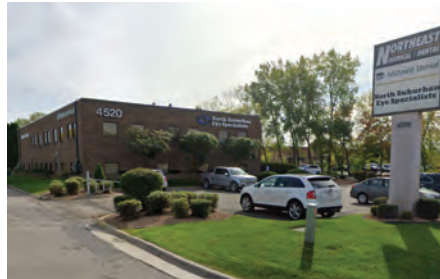
Two-story medical office building adjacent to a gas station and drive-through restaurant building.
