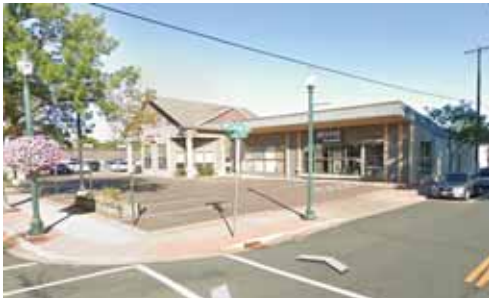
Semi Storefronts in the Core
