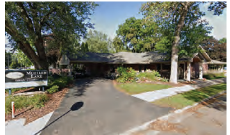
Funeral Home on the edge of the Downtown Edge with residential design characteristics.
