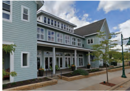
3.5 story apartment building that transitions to 2.5 stories facing the lake. Site includes a mix of residential, commercial, civic and open spaces
