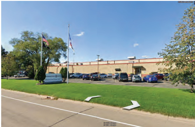
Industrial site with one story building, loading docks in the rear and parking in front.
