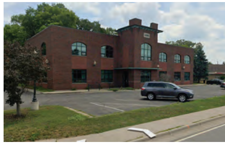
Office buildings in the downtown edge.
