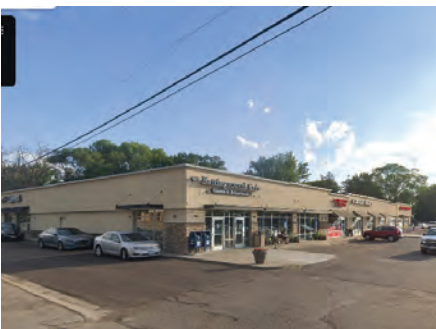
Typical neighborhood restaurant in a multi tenant one story auto oriented building at White Bear Lake and County Rd E
