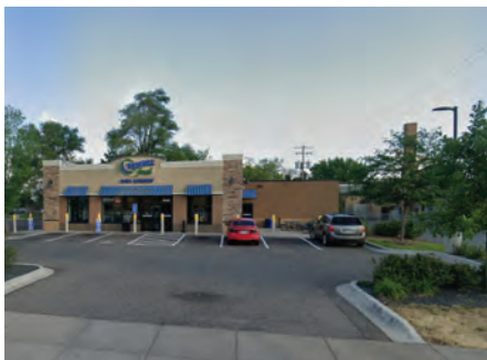
Typical neighborhood service in a one story auto oriented building at White Bear Ave and County Rd E
