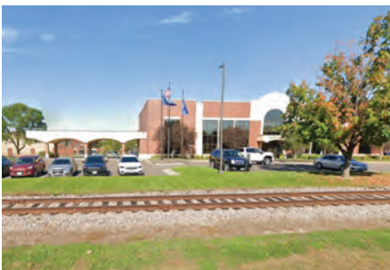
Bank with drive-through.
