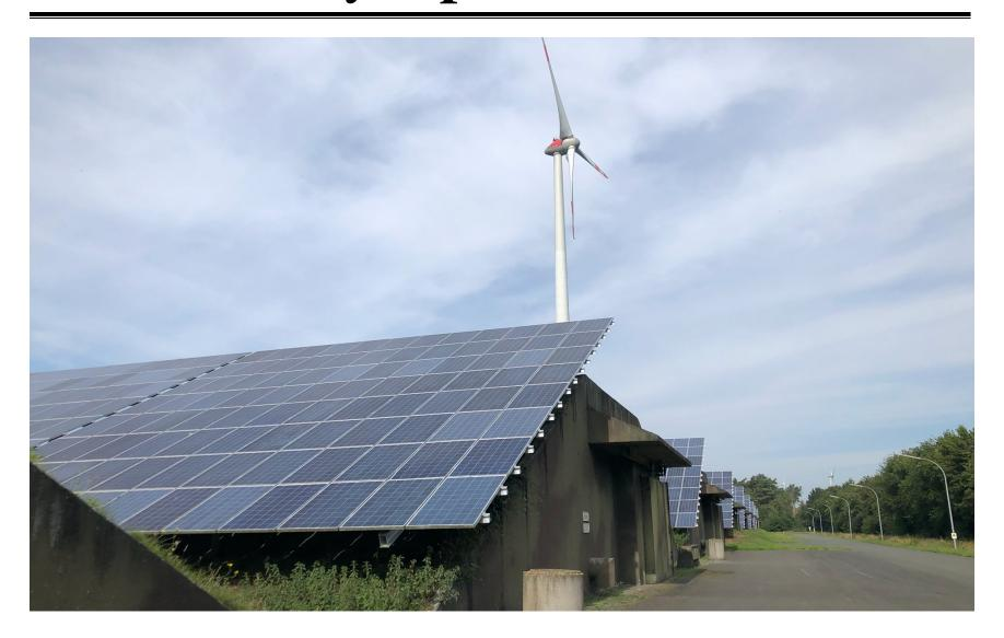
The old military munitions bunkers at the Bioenergie Park have been repurposed to support and cool the solar arrays.
