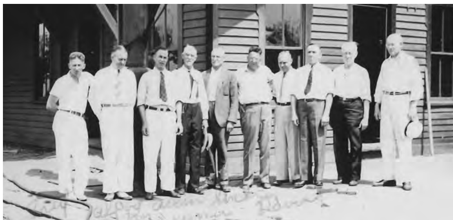
One of the civic organizations that supported the construction of a sewer system in White Bear Lake in the mid-1920s was the members of the White Bear Association, the forerunner of today's Chamber of Commerce. Seen here in 1935 are, left to right, Fred Campbell, Al Podvin, Allen Warner, Captain W.A. Stickley, Charles Davies, Carl Magnuson, Sydney Henkel, Les Palmer, a Mr. Reed, and an unidentified station agent. Photo courtesy of the White Bear Lake Area Historical Society.
