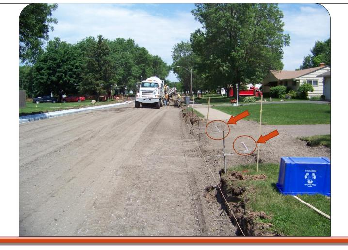
One or two days prior to pouring the curb, crews will mark your driveway openings with small white stakes. These stakes indicate the proposed extents of the curb opening (lowest "drive-able" portion of the curb.
