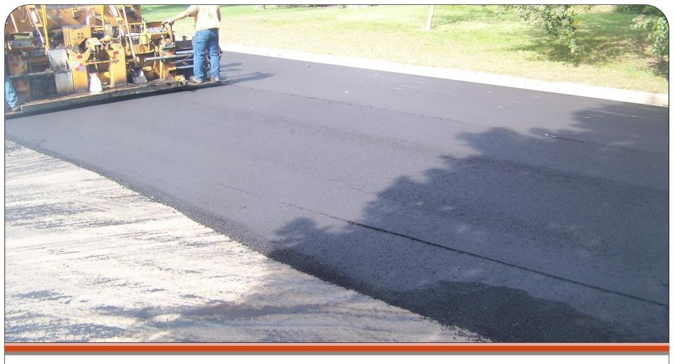
The last step in placement of your new street is laying the final lift of bituminous.
