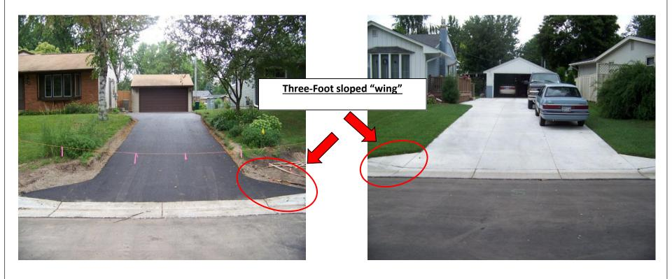
All driveways will also include a three-foot wing on each side which slopes up to match the full height of the curb.
