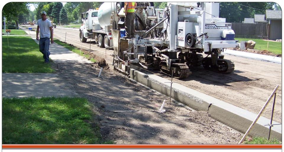
Once the gravel base placement is complete, concrete curb and gutter will be poured. Modern slip-form machines allow this work to proceed very quickly with a single crew, often completing over 5,000 feet per day.
