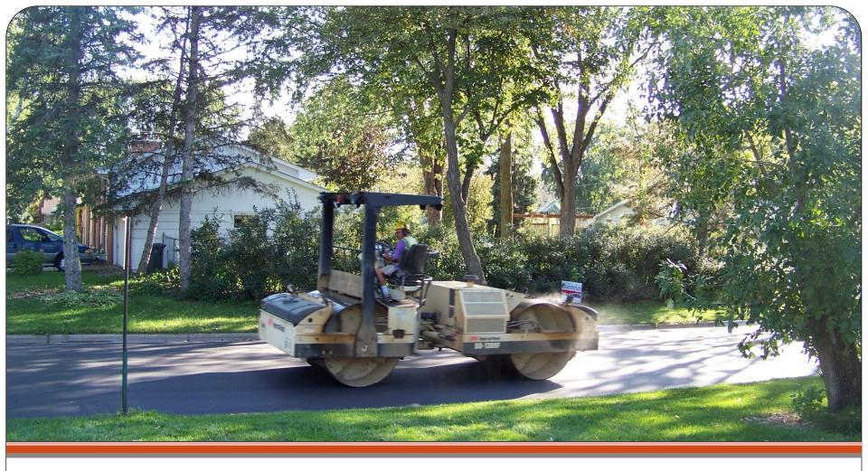
You will not be able to drive on the paved portion of the road for at least two hours or until they have finished rolling the newly paved roads.
