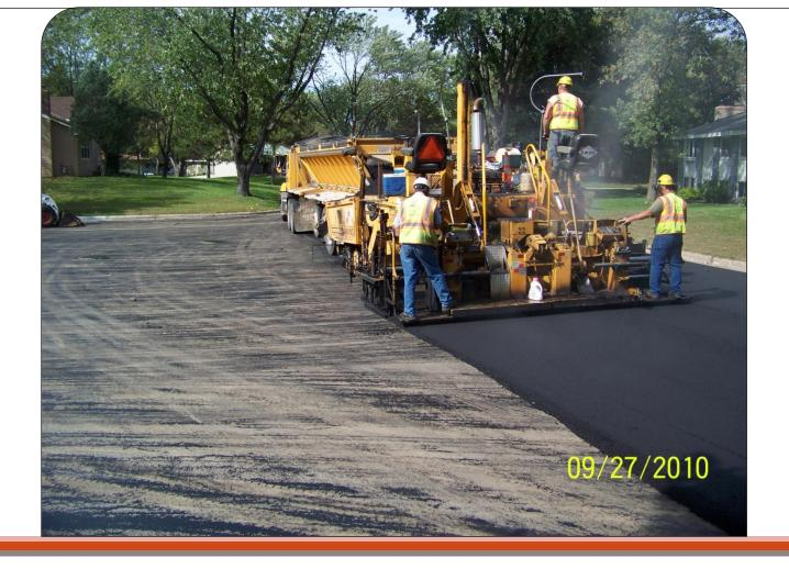
New asphalt is very hot **(approximately 300°F)** when placed. Parents should keep children and pets a safe distance away from the new pavement until it cools.
