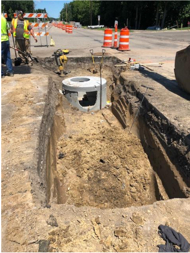
Storm Sewer Installation – Median (Centerville Road)
