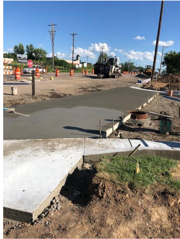
Driveway Installation – Cub Foods
