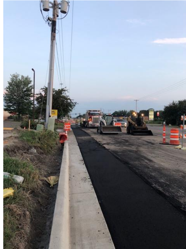
Lane Widening – East Side (Centerville Road)
