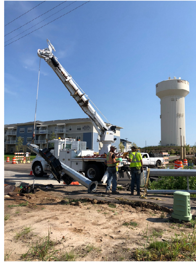
Signal Pole Installation – Centerville Road
