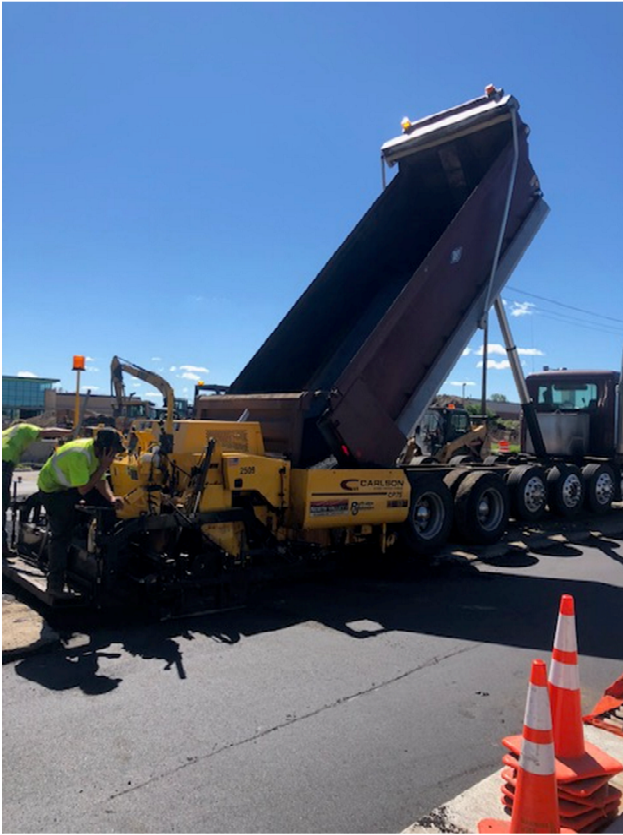
Shoulder Paving – Centerville Road
