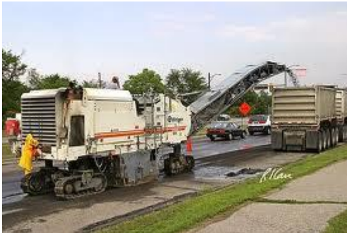
Milling Machine in operation
