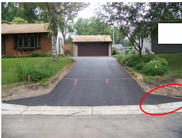
Three-Foot sloped “wing”
