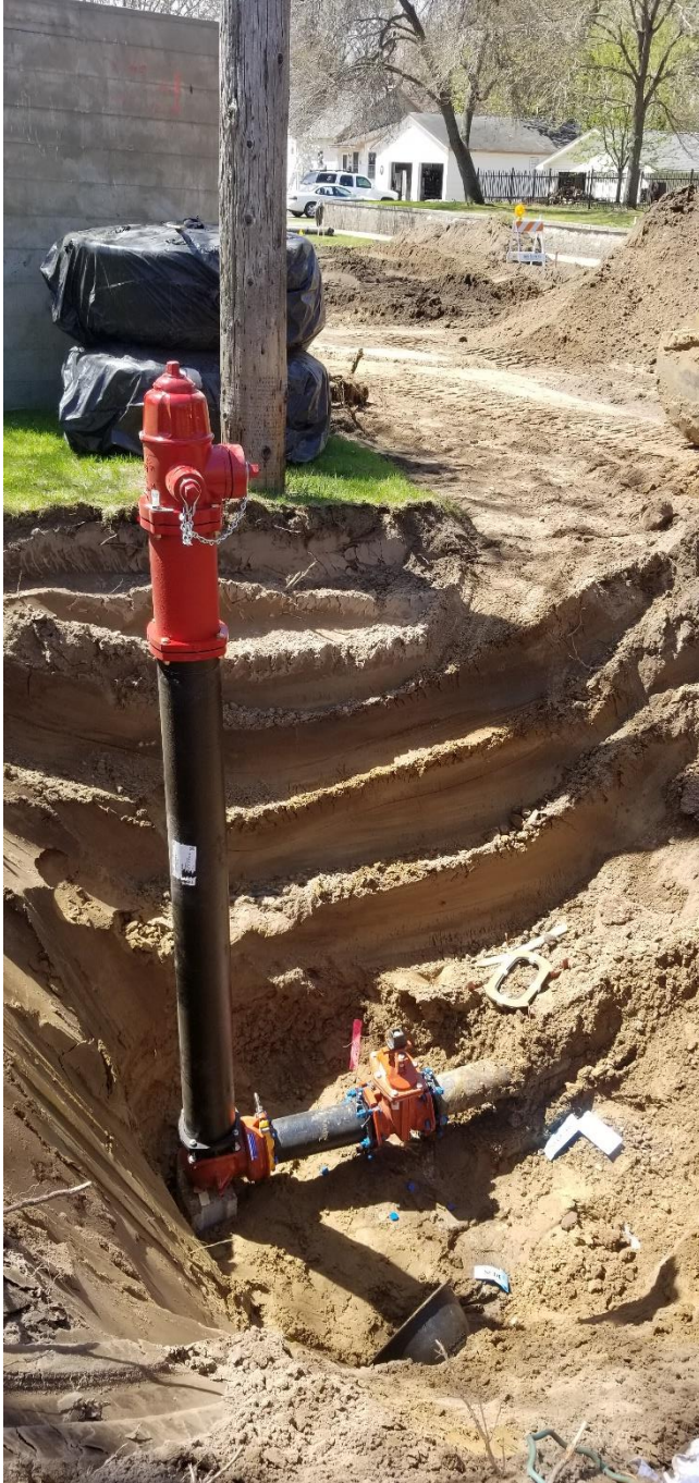
Hydrant replacement at 6 th Street and Johnson Avenue
