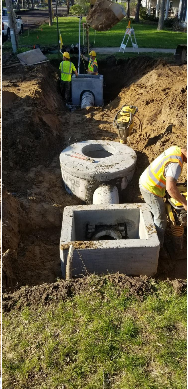
Storm sewer installation at 6 th Street and Johnson Avenue
