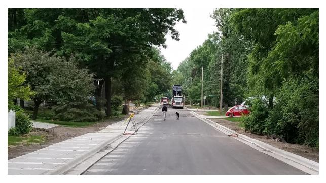
11<sup>th</sup> Street is nearly complete. Following a few more construction activities, the Contractor will return to place the final lift of asphalt pavement. Until then, please drive very slow and avoid the protruding manhole castings.
