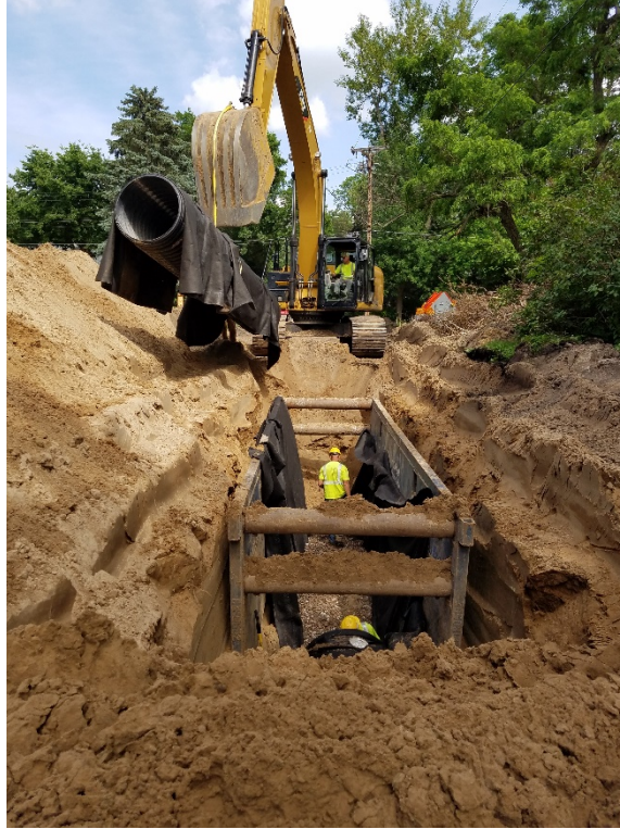
Workers place a new storm water treatment system beneath 8 th Street.
