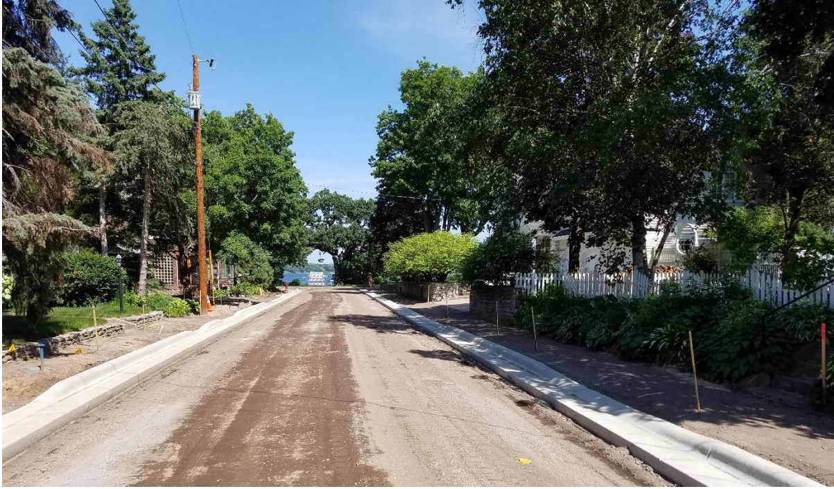
New curb and gutter along 9 th Street.
