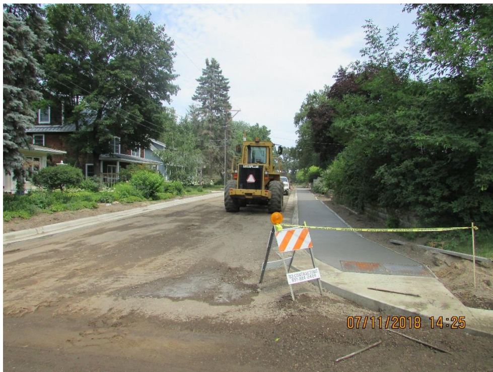
Newly constructed sidewalk along 9 th Street at Johnson Avenue.
