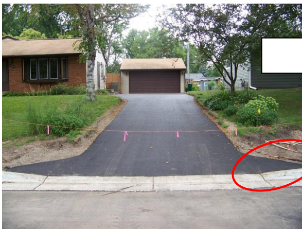
Three-Foot sloped “wing”
