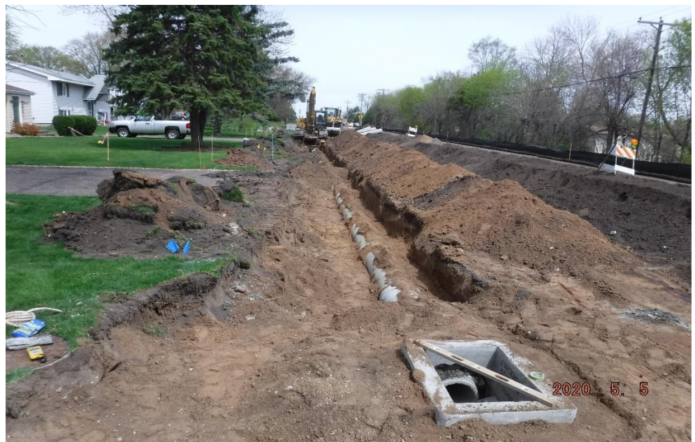
Storm sewer installation
