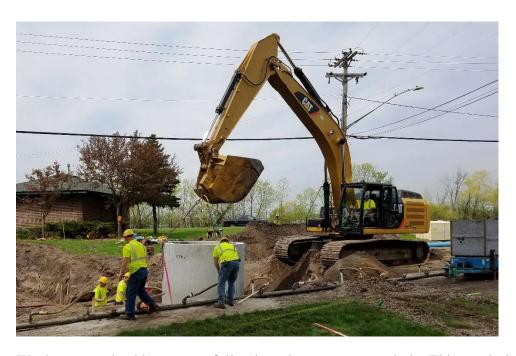
Workers use a backhoe to carefully place the concrete manhole. This manhole will allow personnel to access and operate the new sanitary sewer forcemain.
