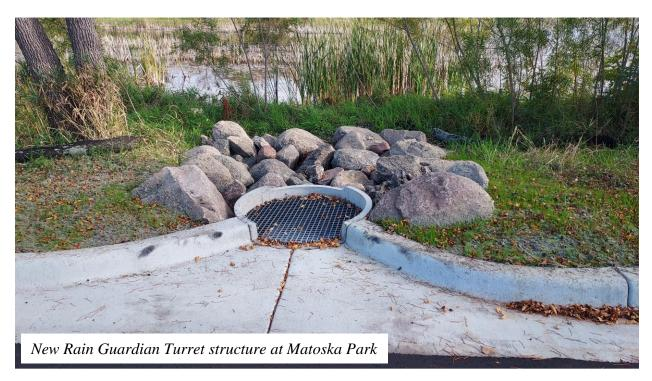
A third Rain Guardian Turret structure was install this summer as part of the Lakewood Hills Park parking lot rehabilitation project. This Turret will serve as a pretreatment structure for a future raingarden that is proposed to be constructed in 2022. The City is currently working with the Ramsey Washington Metro Watershed District (RWMWD) on the design of the raingarden, and will apply for a RWMWD cost share grant in early 2022 to help cover the cost of raingarden construction.
