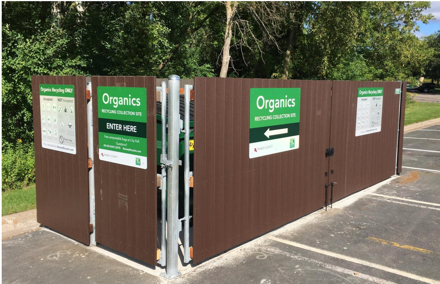
Organics Dumpster Enclosure
