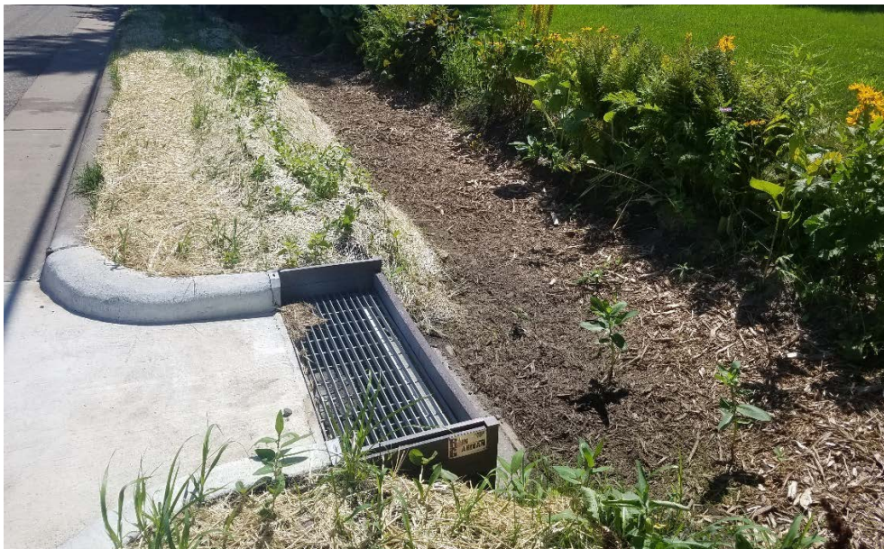
Curb cut and Rainguardian pretreatment structure
