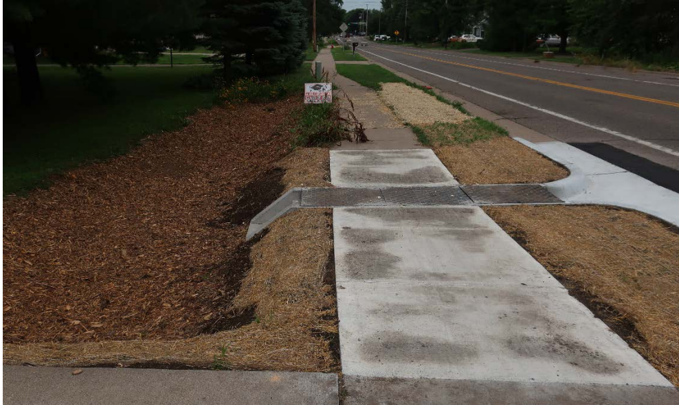
Curb cut and Rainguardian 'Foxhole' pretreatment structure (for use under sidewalks)
