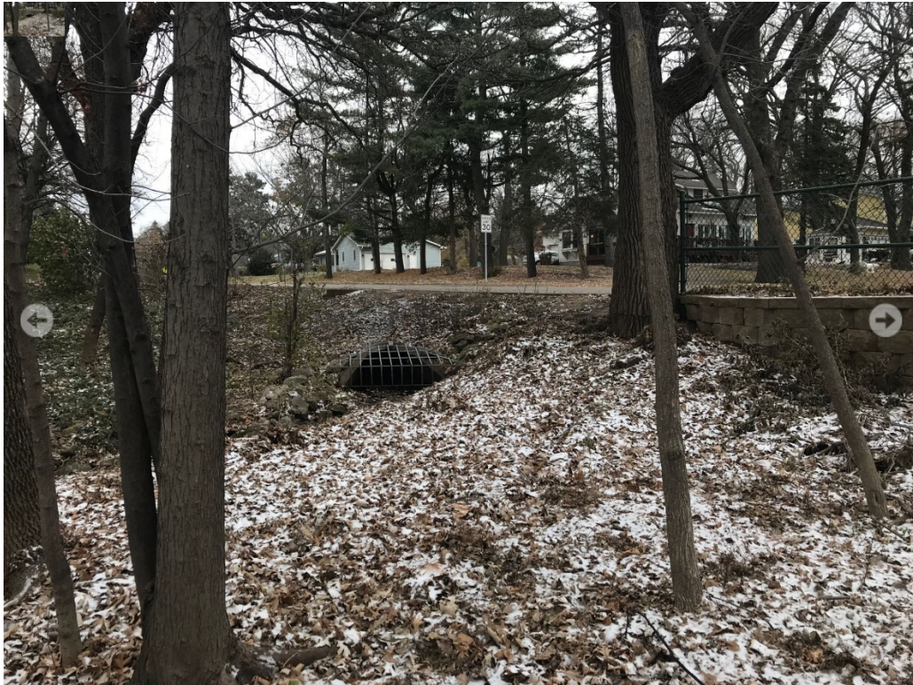
Before: looking southeast towards 4 th Street (photo compliments of VLAWMO)
