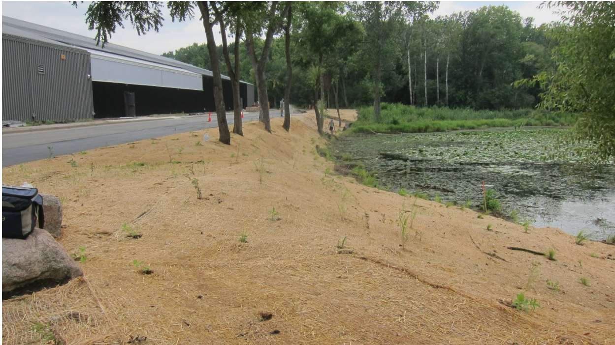
August 23, 2018 – Seeding and erosion control blanket
