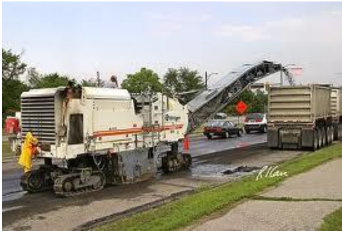
Milling Machine in operation
