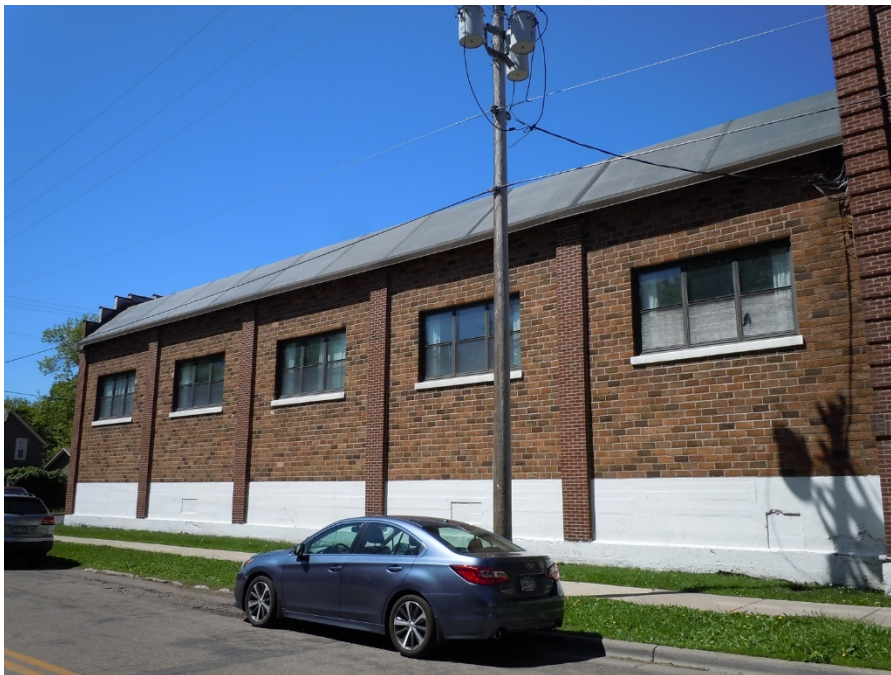
FIGURE 16. EAST SIDE OF DRILL HALL, LOOKING SOUTHWEST
