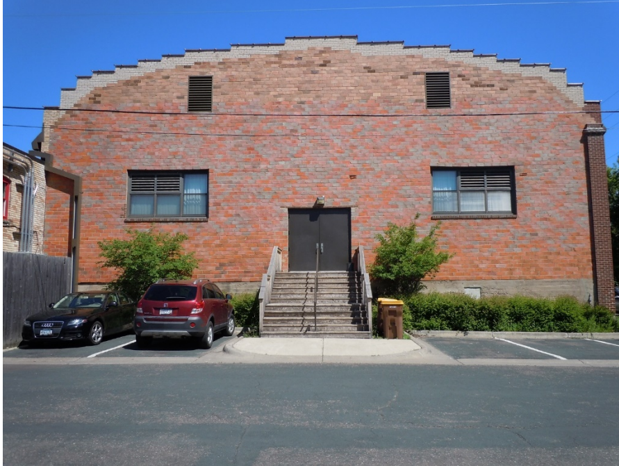
FIGURE 17. SOUTH END OF DRILL HALL, LOOKING NORTH
