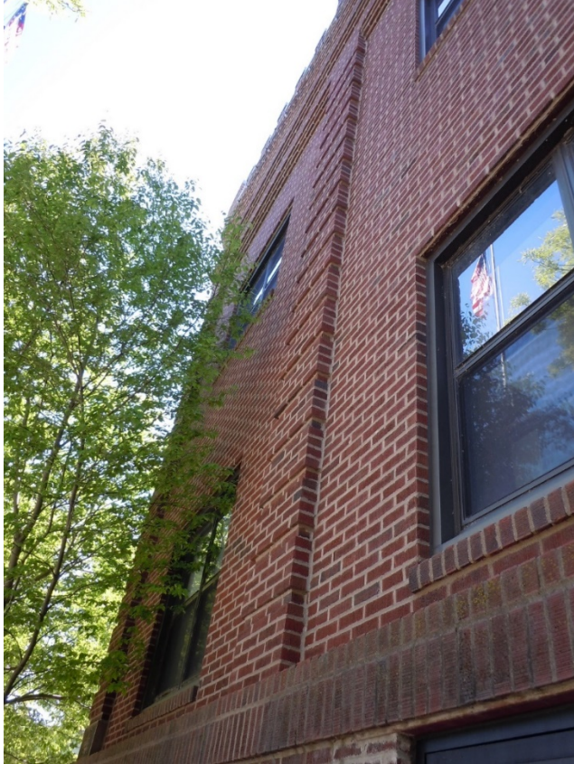
FIGURE 13. DETAIL OF PILASTER DIVIDING EAST AND CENTRAL BAYS, LOOKING EAST-SOUTHEAST
