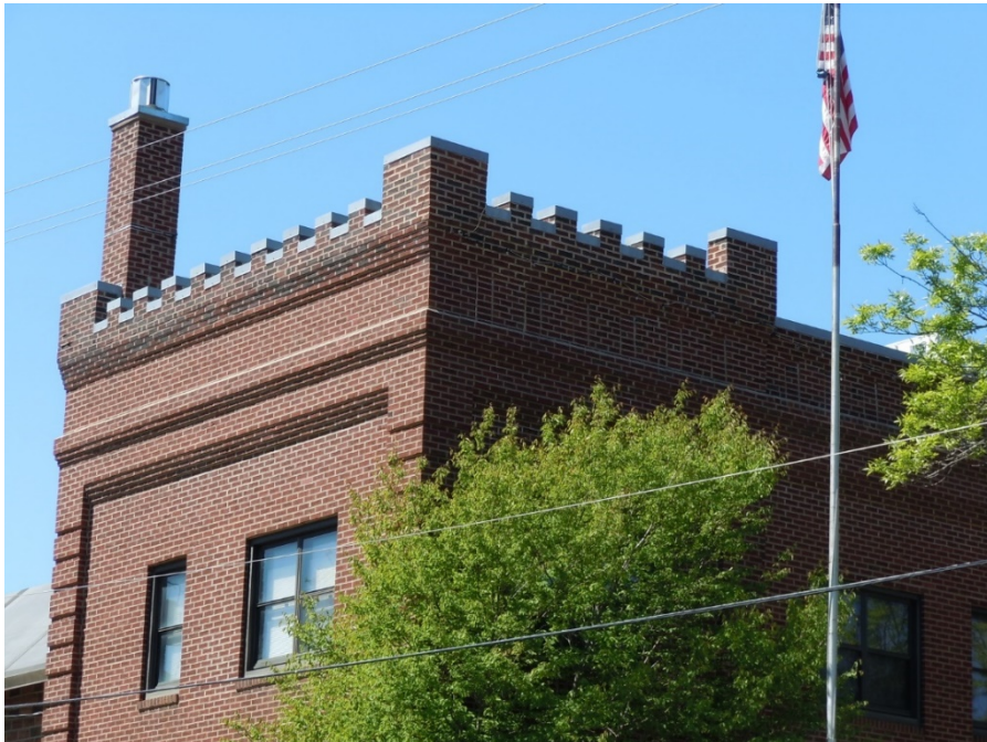
FIGURE 14. DETAIL OF UPPER NORTHEAST CORNER, LOOKING SOUTHWEST
