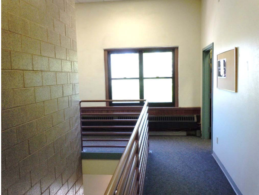
FIGURE 23. SECOND FLOOR WALKWAY, LOOKING NORTH
