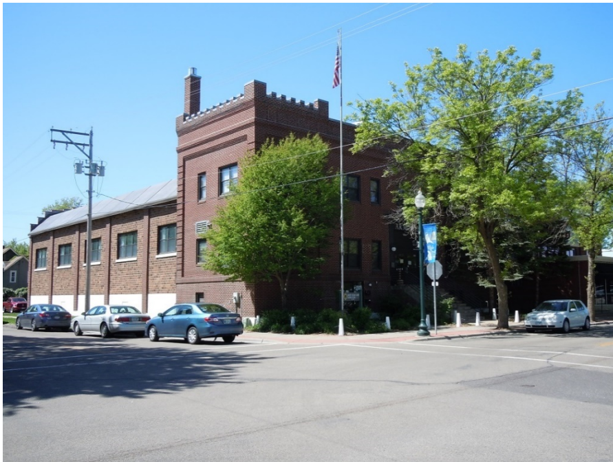
FIGURE 10. WHITE BEAR LAKE ARMORY, LOOKING SOUTHWEST
