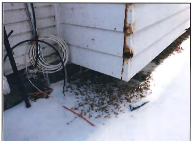
6 Overhang from foundation on existing house at 4556 Highway 61 is approx. 2'-4".
