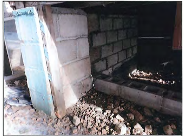
8 Existing foundation at 4556 Highway 61.
