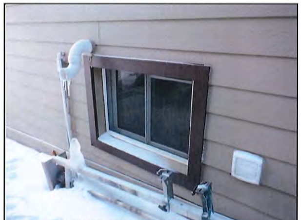
12 Existing conditions along north side of 4552 Highway 61.
