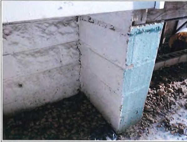
7 Existing foundation at 4556 Highway 61.
