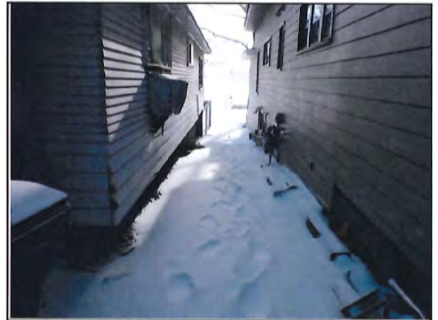
2 View between existing structures looking east.
