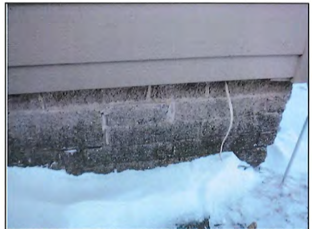
10 Existing garage foundation wall on north side of 4552 Highway 61.
