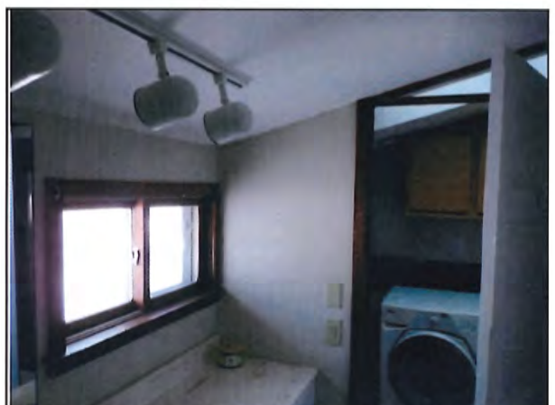
18 Existing conditions along north side of upper apartment.
