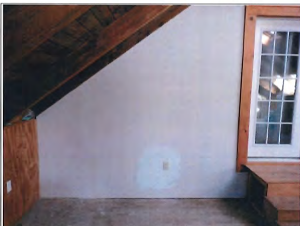
17 Existing conditions along north side of upper level loft area over garage.
