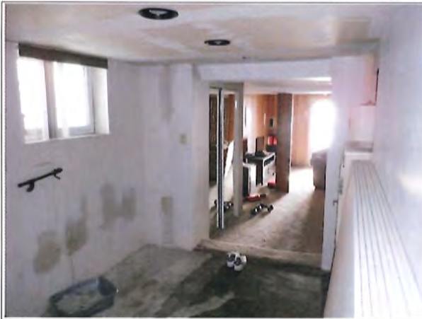
13 Existing conditions along north basement wall. Foundation concealed.
