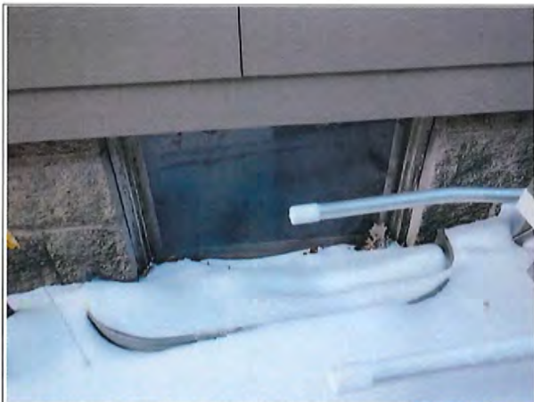
11 Existing north foundation wall at 4552 Highway 61.
