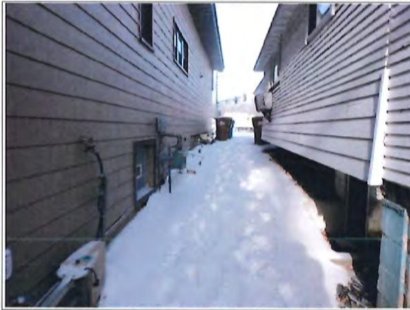
3 View between existing structures looking west.
