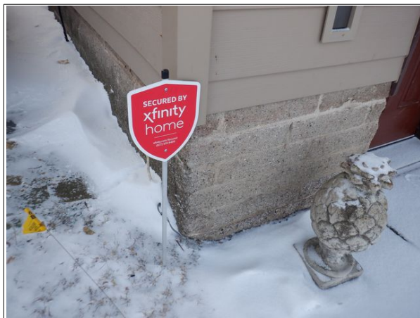
9 Existing garage foundation wall at northwest corner of 4552 Highway 61.
