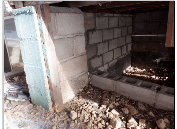
8 Existing foundation at 4556 Highway 61.
