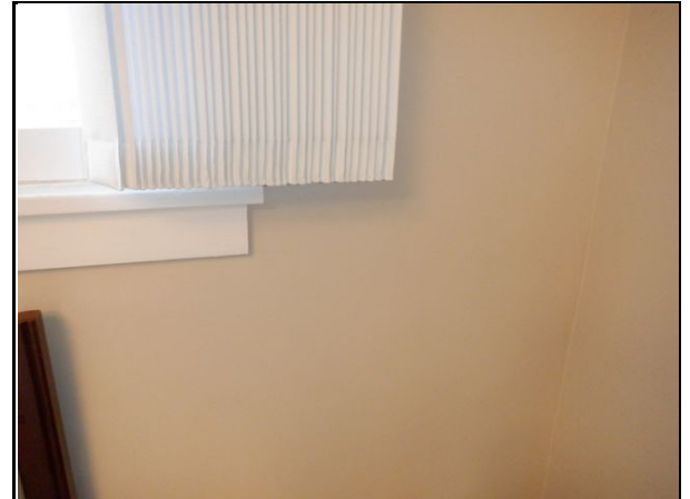
16 Existing conditions at main level bedroom on north side of house.
