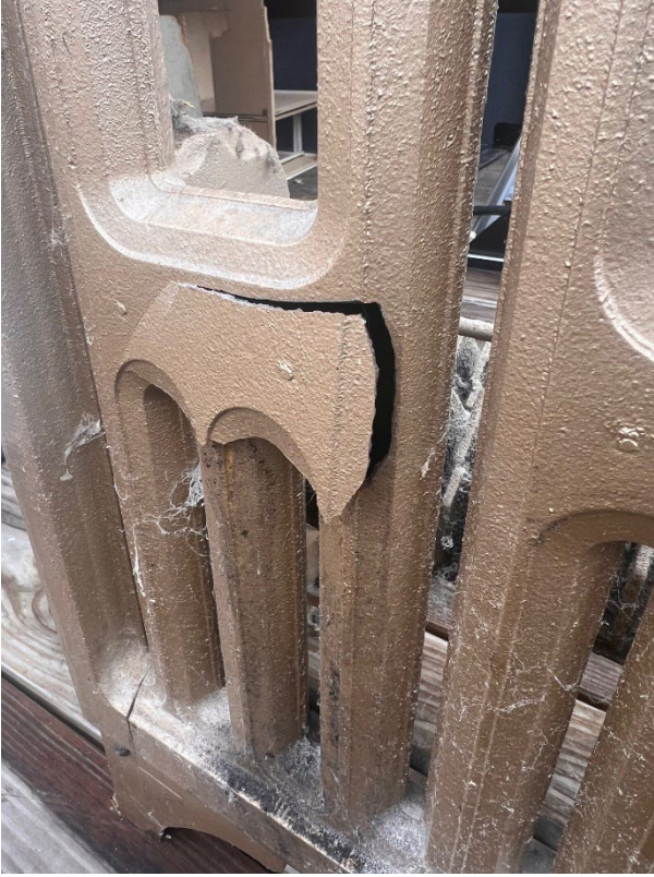
7- Radiator piping burst
