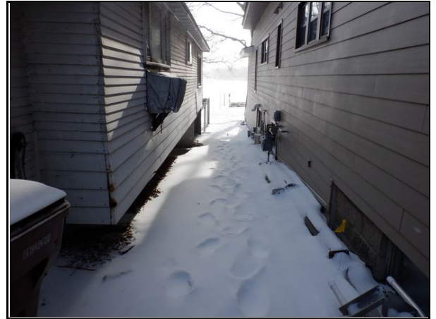
2 View between existing structures looking east.
