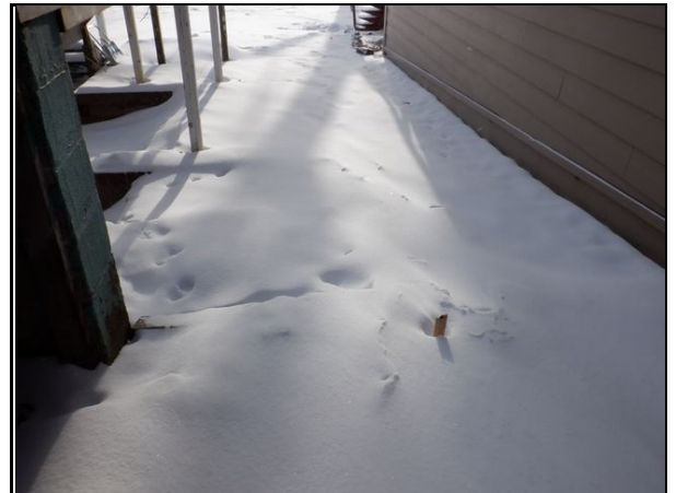
4 View between existing structures looking east.
