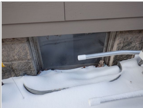
11 Existing north foundation wall at 4552 Highway 61.
