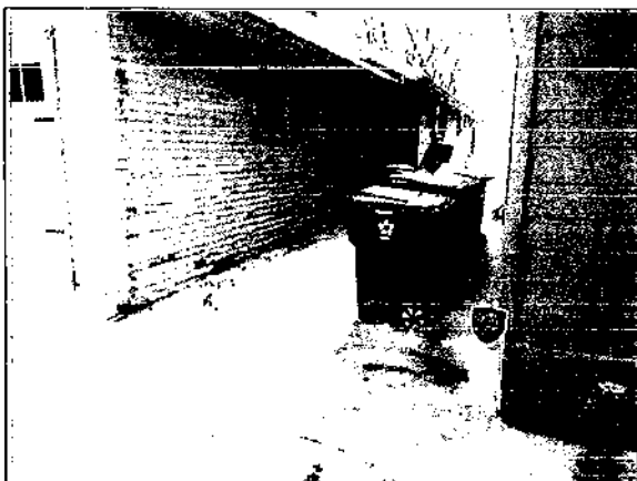
1 View of area between structures. (4552 Hwy, 61 on right, 4556 Hwy, 61 on left). Approx. 9.5'
