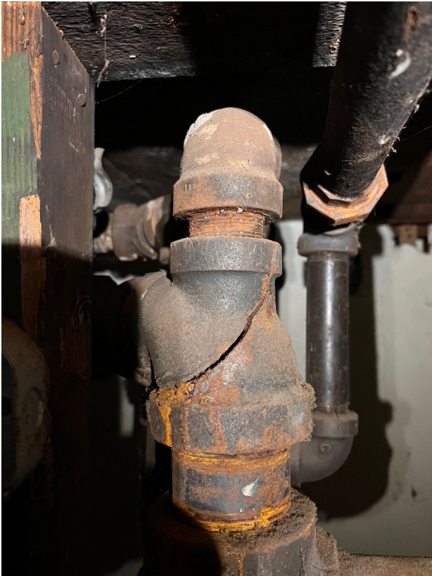
7- Radiator piping burst
