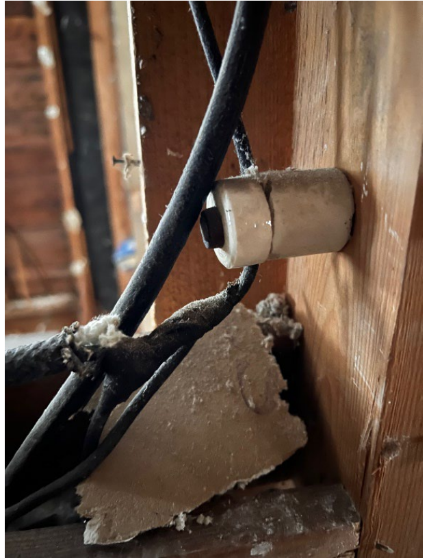
3- Electrical 3- knob & tube cloth wiring
