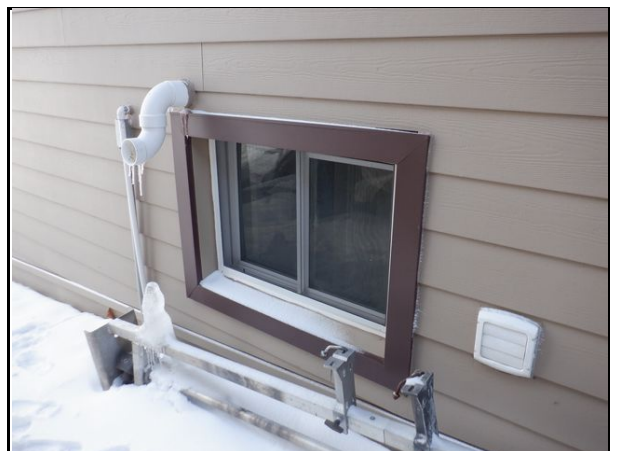
12 Existing conditions along north side of 4552 Highway 61.
