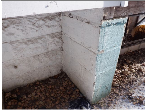
7 Existing foundation at 4556 Highway 61.
