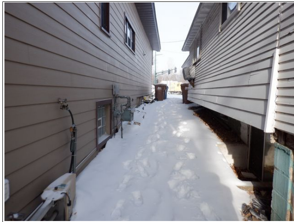
3 View between existing structures looking west.
