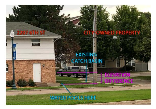
2. Water falling on the City-owned property sheds Southeast until it hits the 2207 foundation wall, where it tends to pool underground, saturating the soil. This exerts hydrostatic pressure on the 2207 foundation wall.
