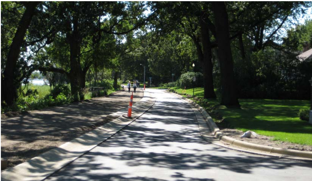
Lake Avenue roadway and trail under reconstruction, Summer of 2007.
