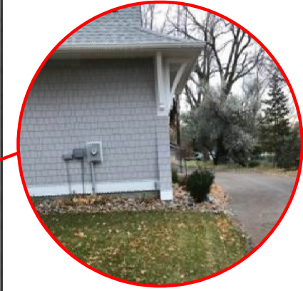
#4304 ~2 FEET (ADJACENT NEIGHBOR TO THE SOUTH)
