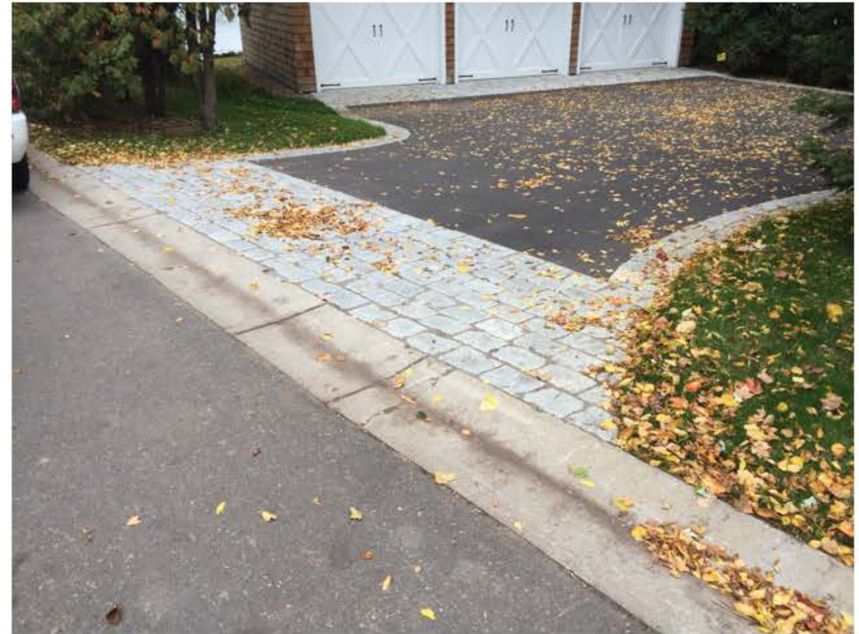
Gate placement at asphalt/stone junction to allow ideal access and shortest span.
