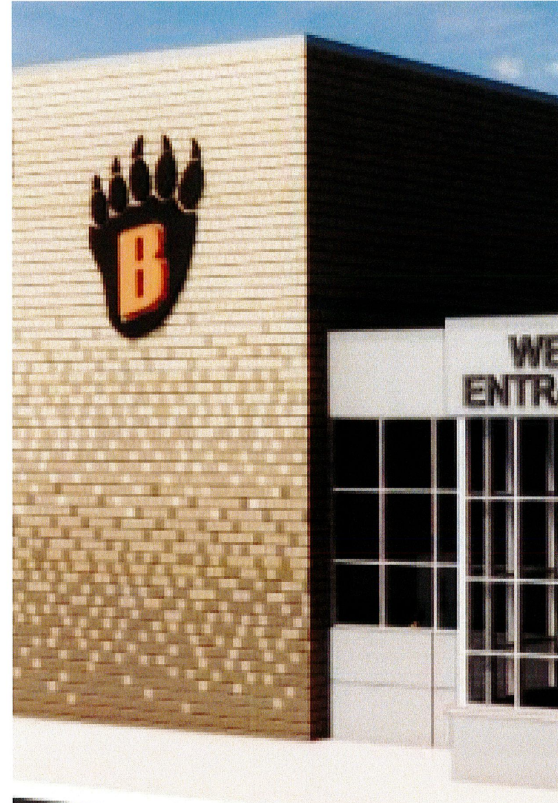
GYM ADDITION (CURRENTLY UNDER CONSTRUCTION)
