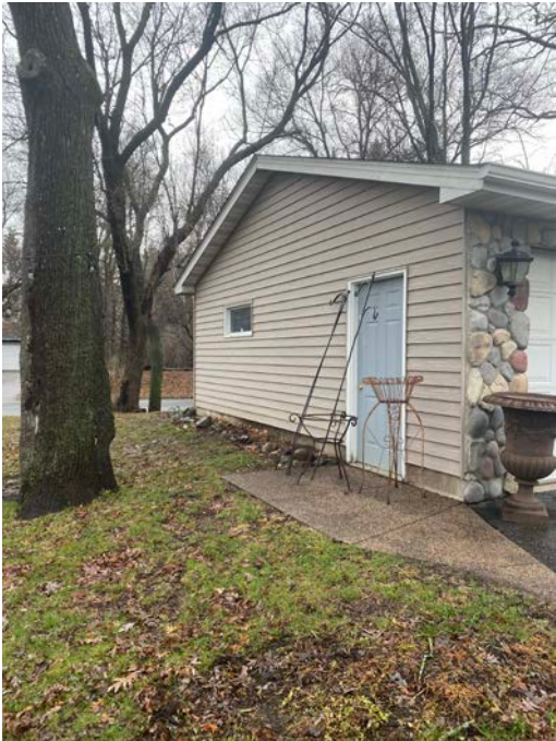
West side of existing garage:
