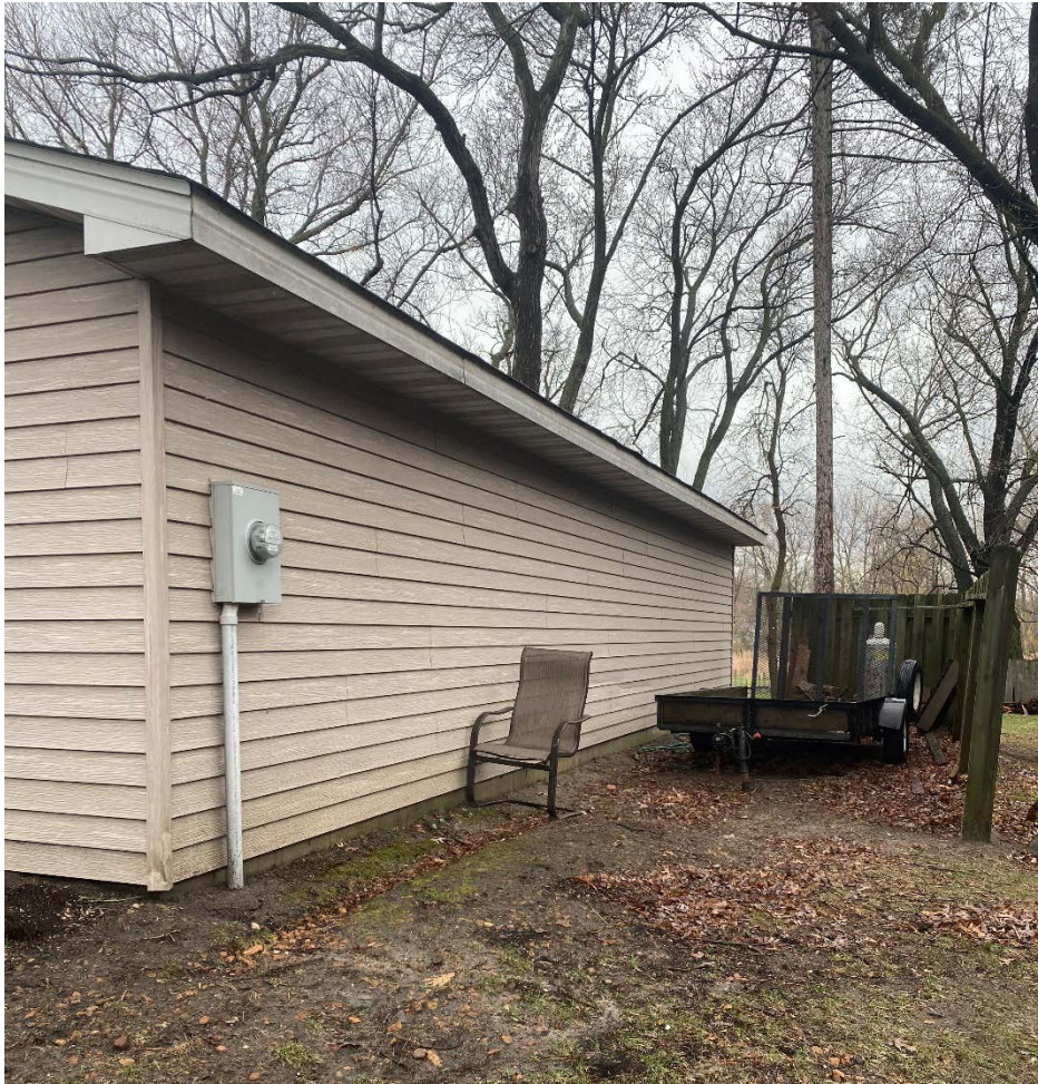
Back (north) side of existing garage:
