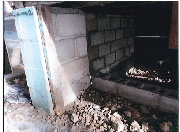
8 Existing foundation at 4556 Highway 61.
