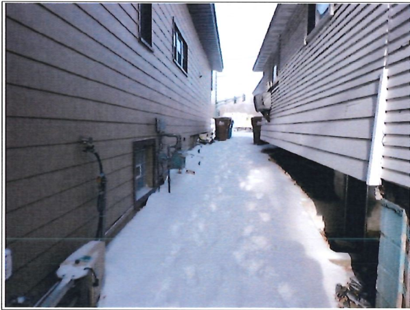
3 View between existing structures looking west.
