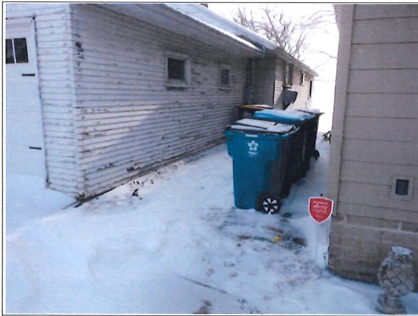
1 View of area between structures. (4552 Hwy, 61 on right, 4556 Hwy. 61 on left). Approx. 9.5'
