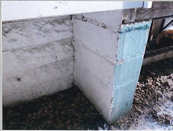
7 Existing foundation at 4556 Highway 61.
