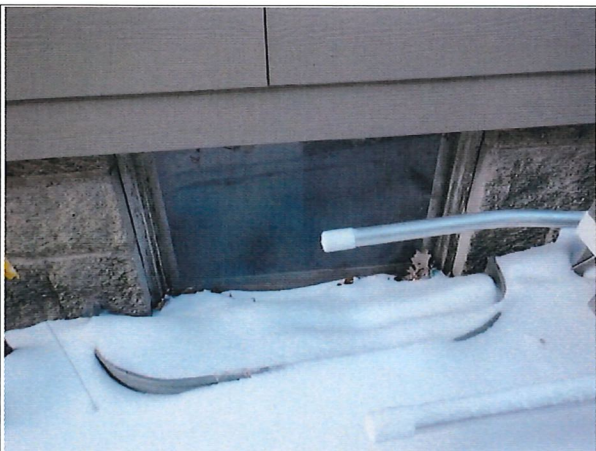
11 Existing north foundation wall at 4552 Highway 61.
