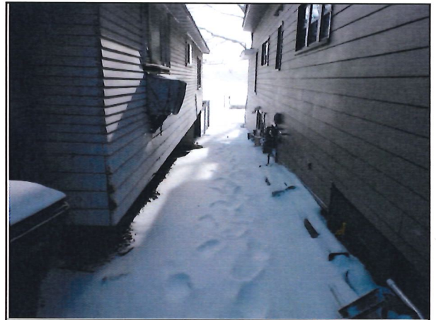
2 View between existing structures looking east.
