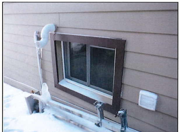
12 Existing conditions along north side of 4552 Highway 61.
