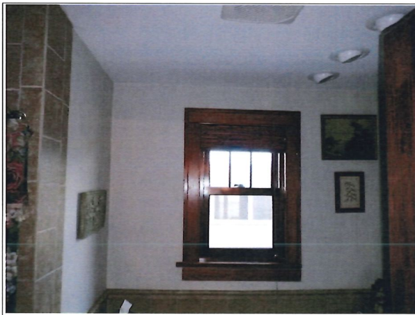
15 Existing conditions at main level bathroom on north side of house.
