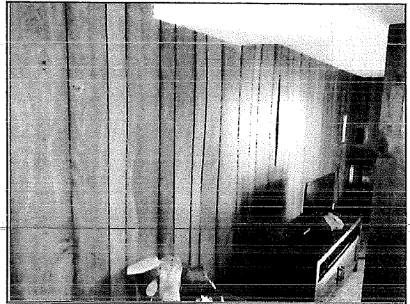
14 Existing conditions along north basement wall. Foundation concealed by paneling.
