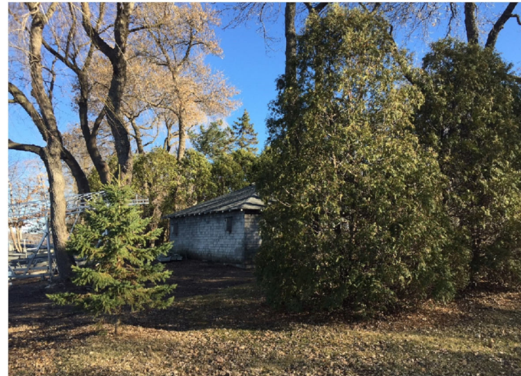
Garage Side/Rear from Street side
