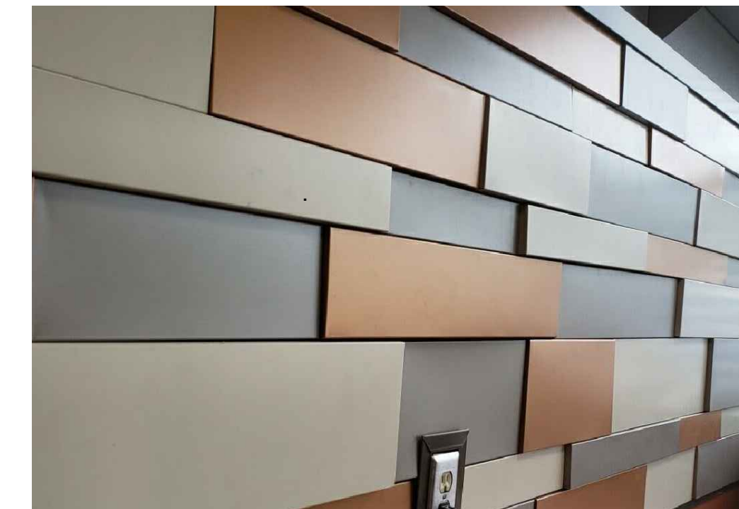
5 EXAMPLE OF EXTERIOR METAL PANEL ENCLOSURES NOT TO SCALE (FOR COURTYARD ENCLOSURE TRAINING)
