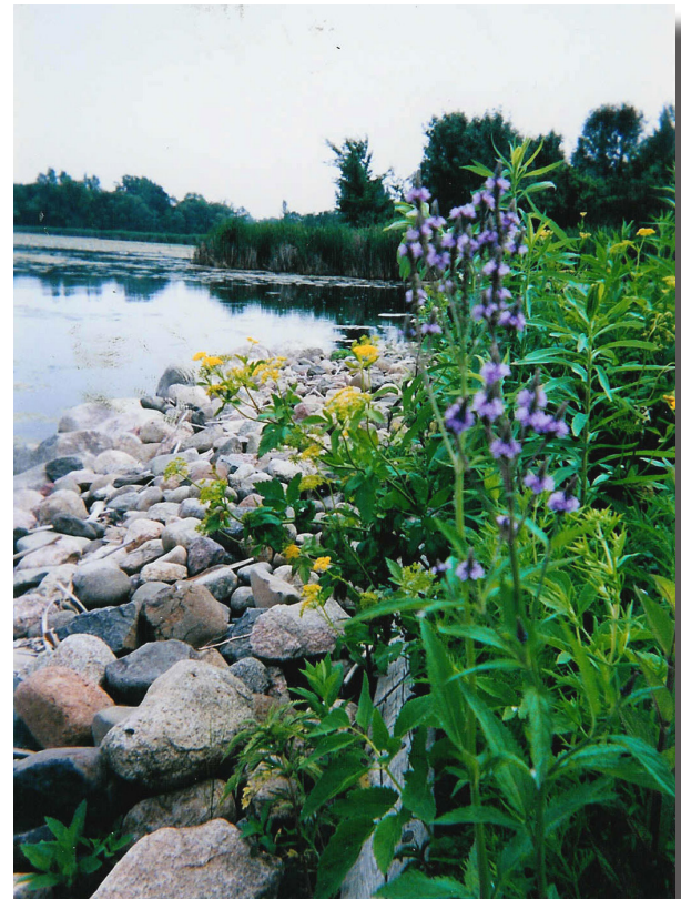
Shoreline stabilized with riprap and enhanced with a vegetative buffer.
